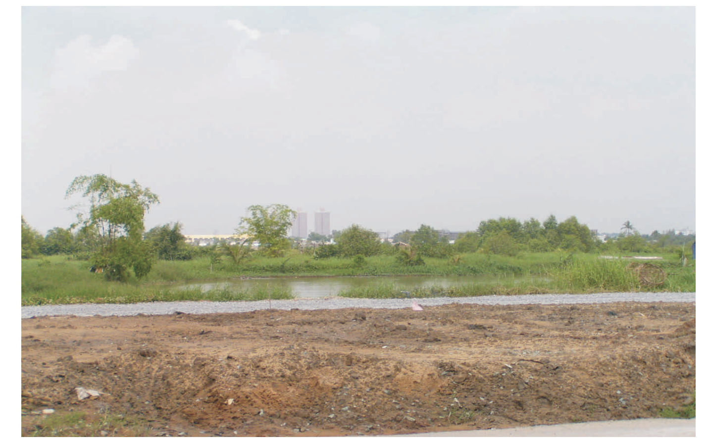
Upgrading the road along fish ponds
