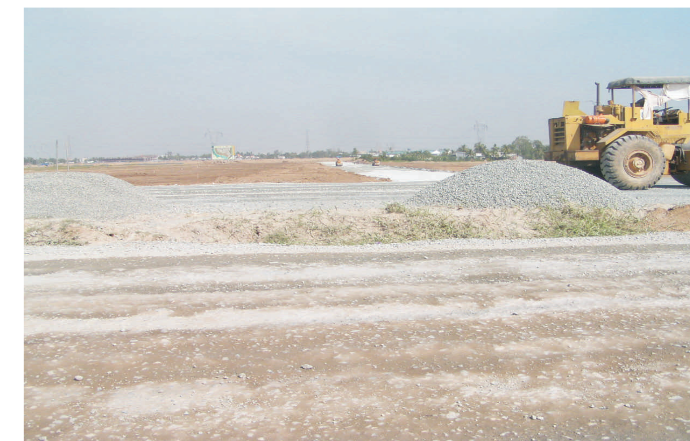
Construction site of residential area
