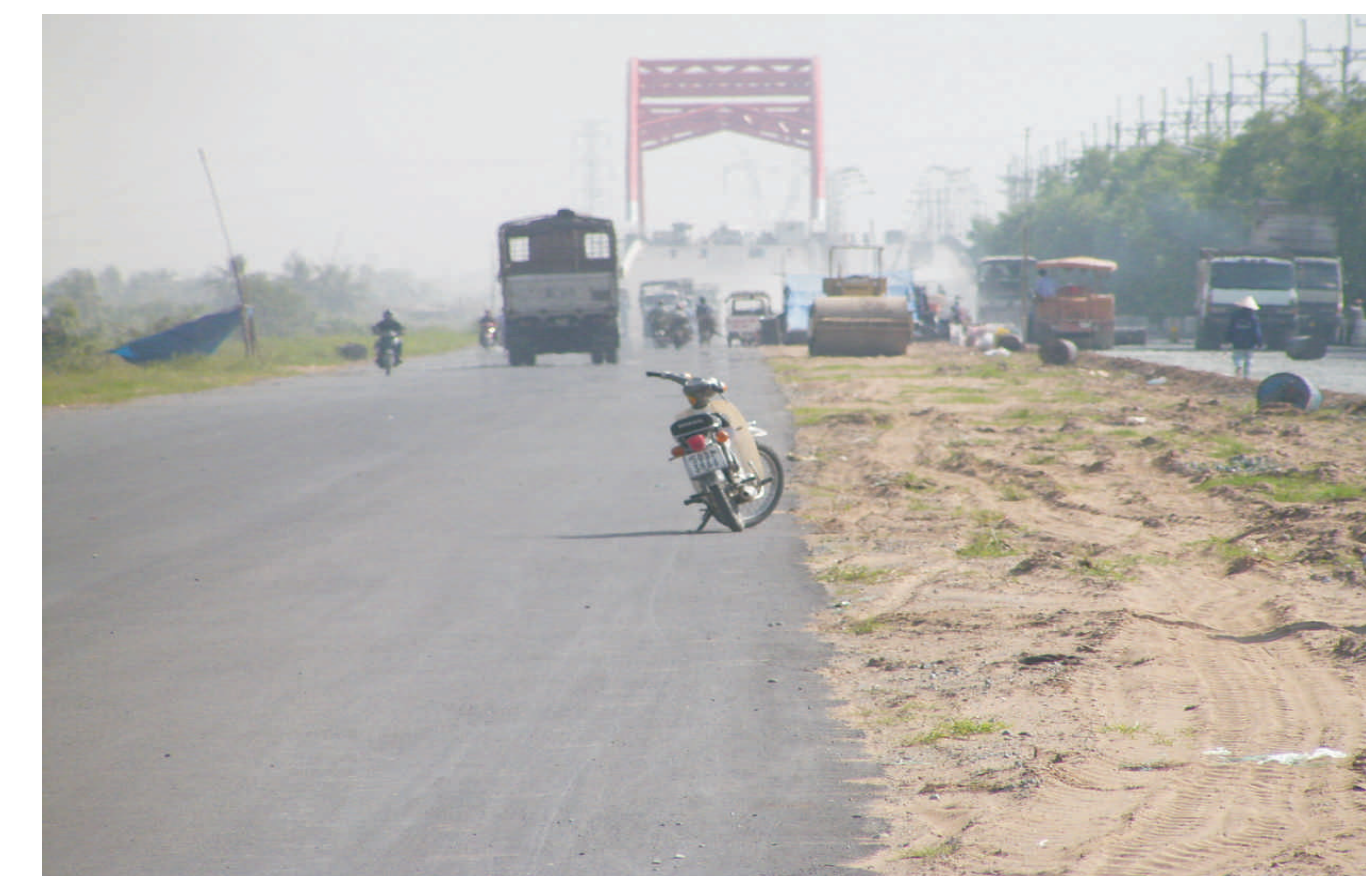
Construction site of the new bridge on Nguyen Van Linh highway
