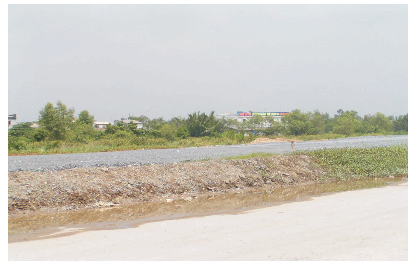
New road built along fish ponds
