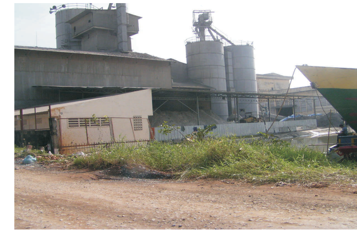
Binh Dien cement factory, Tan Kien Commune, Binh Chanh District
